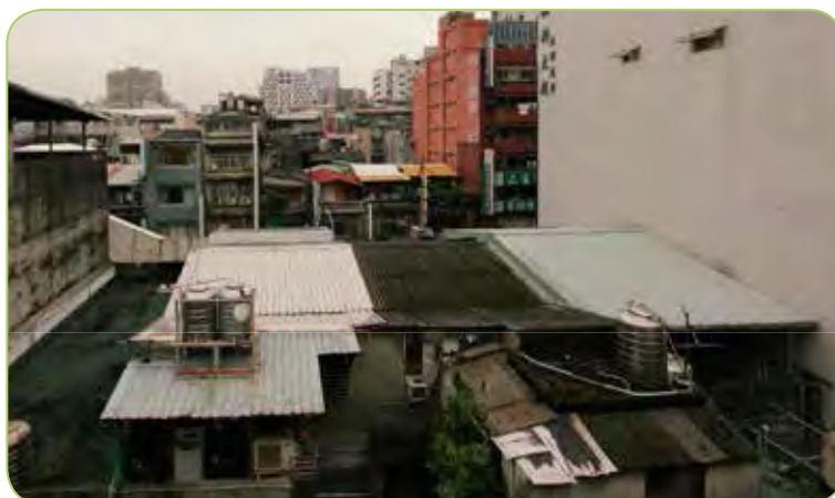
Existing Rooftop Condition
