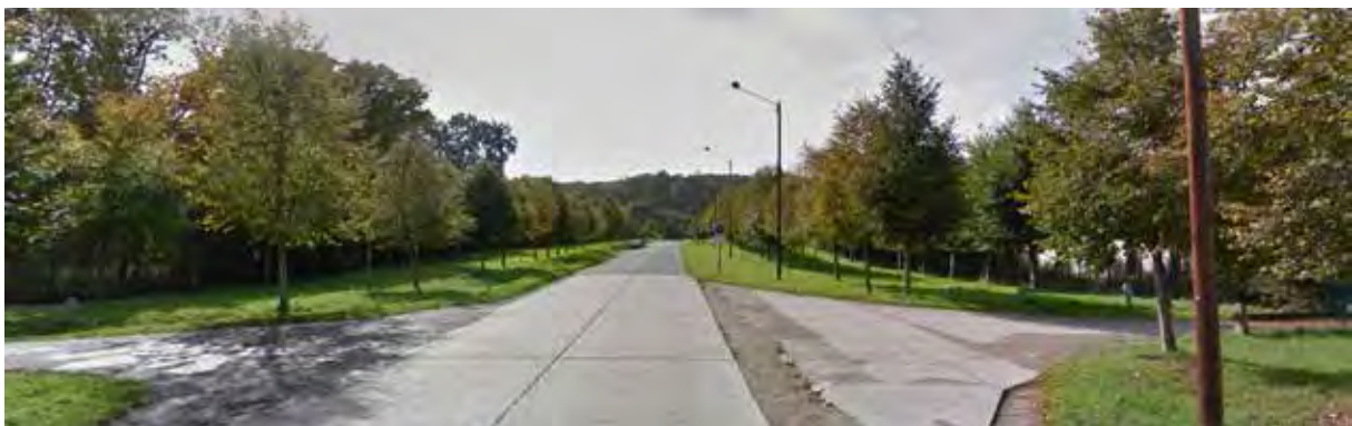
Figure 4.3.6 View of the La Cité du Soleil
