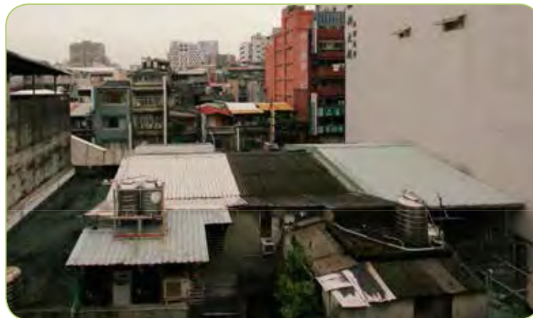
Existing Rooftop Condition
