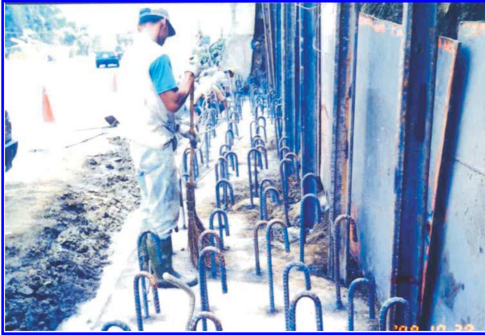
Fig. 8. Shearing reinforcement at construction joint.
