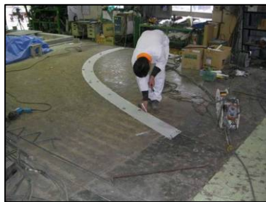
桁架曲線落樣
