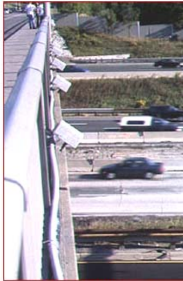
Testing the performance of traffic detectors
